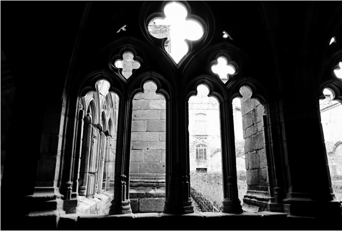
Figure 33 – A horizontal shot of the church archways.
